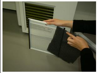
Filter is held with the filter fixing plate. Remove the filter and wash or remove dust with an electric cleaner with the filter attached.
